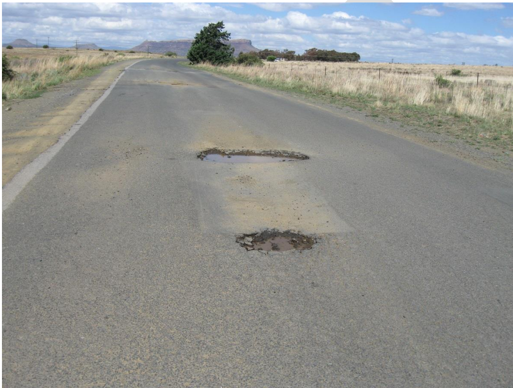
Photograph 8: Potholing of the main access road from R26 to Zastron. Reconstruction will be necessary in places.
