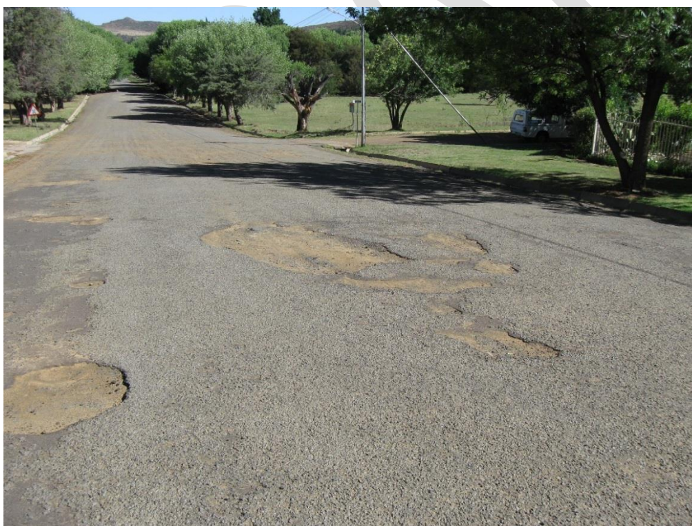
Photograph 10: Many streets in Zastron are breaking up. Urgent maintenance is required before the situation gets worse and major reconstruction becomes necessary.
