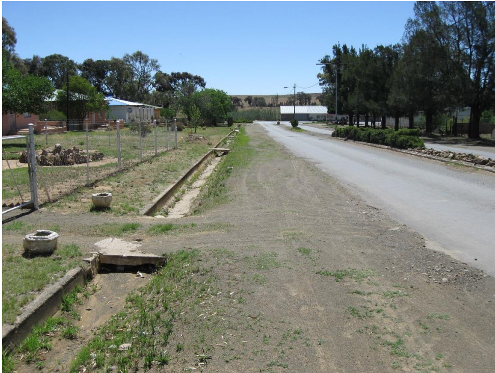
Photograph 4: This street in Rouxville needs shaping of the verge in order to facilitate proper drainage.
