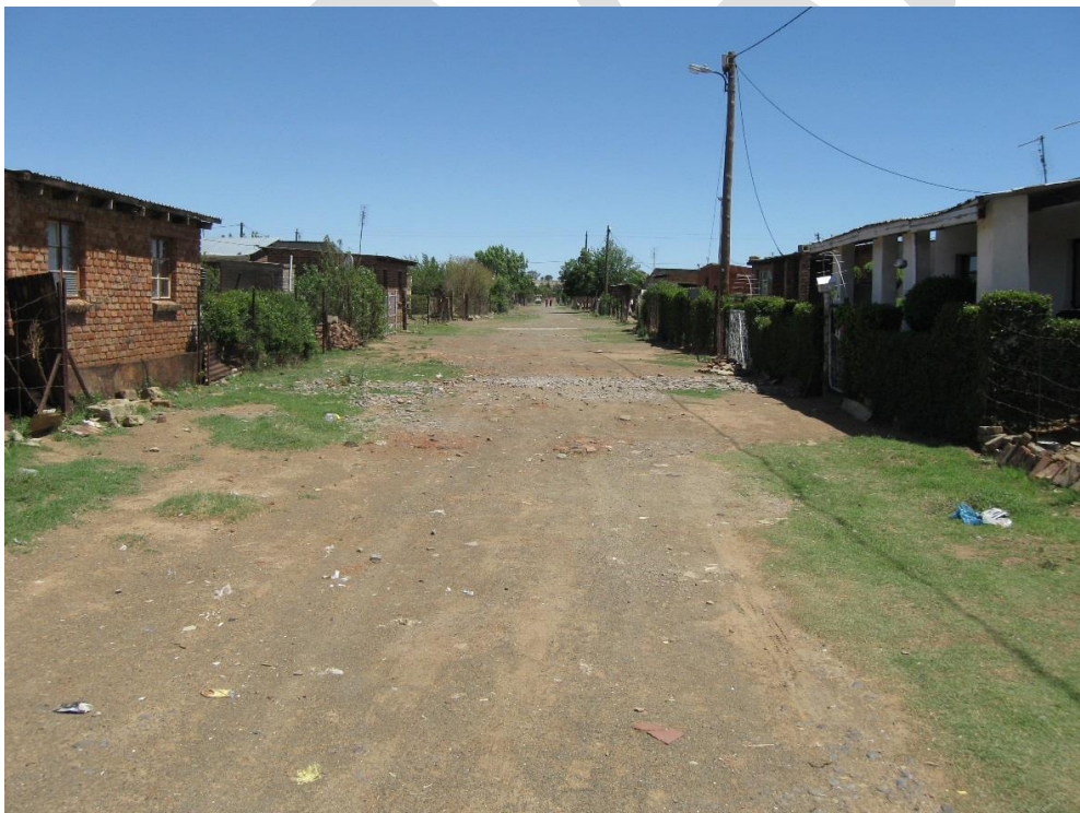
Photograph 7: This gravel track in Roleleathunya is eroded and needs to be gravelled and properly shaped in order to facilitate efficient drainage.
