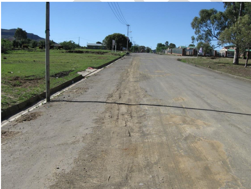
Photograph 12: The main access road between Zastron and Matlakeng can no longer be patched and reconstruction is required.
