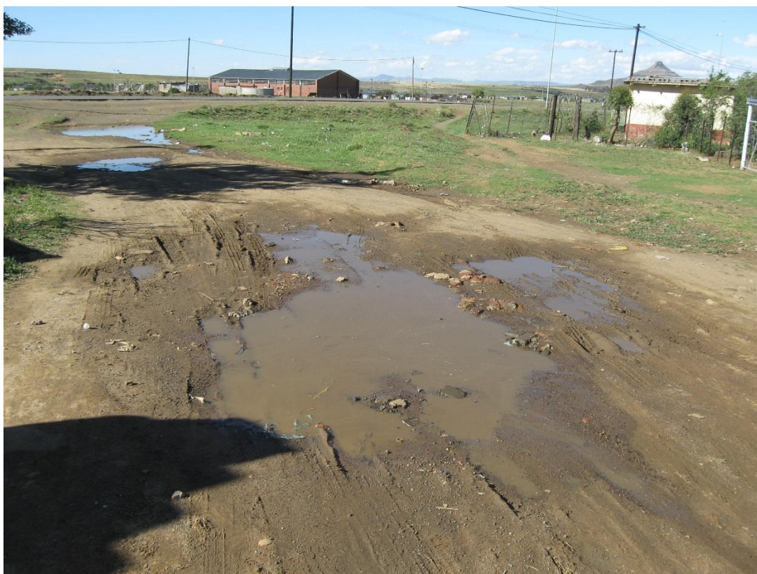
Photograph 8: Example of non-existent stormwater drainage in Matlakeng. This problem is common in the townships and can be alleviated by re-gravelling and shaping the road and constructing lined drains.
