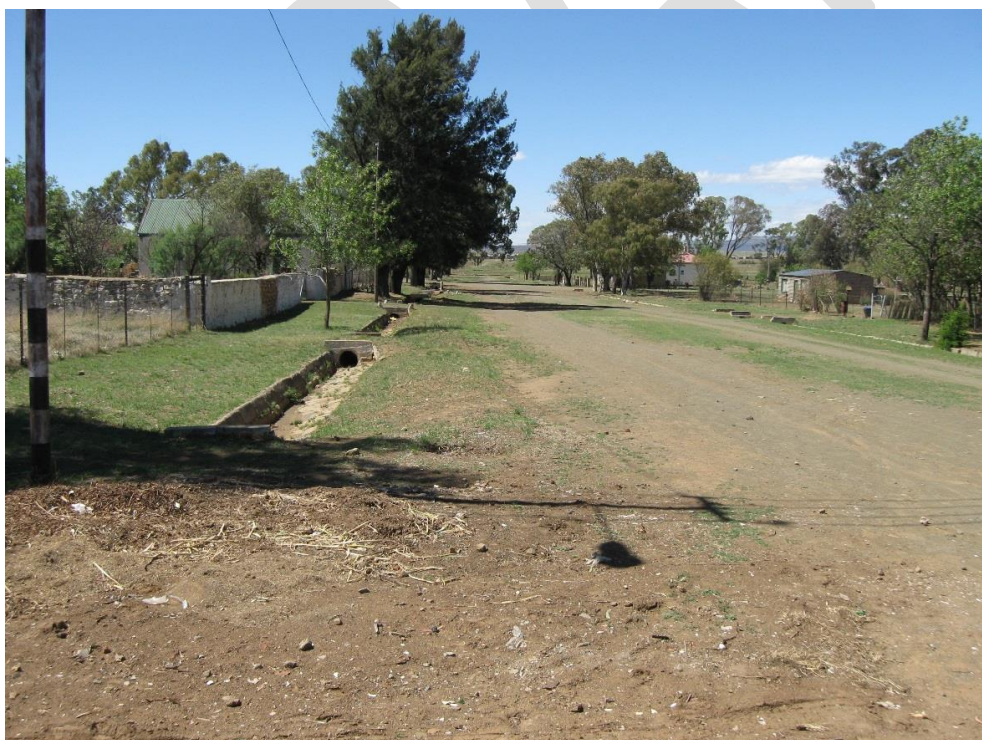
Photograph 6: Street in Rouxville. The verge needs to be trimmed and shaped in order to facilitate proper drainage.
