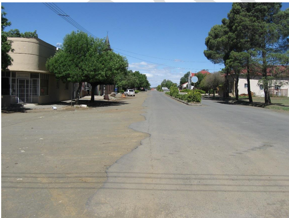
Photograph 5: Edge break at a surfaced road in Rouxville. This requires urgent repair in order to prevent further damage.
