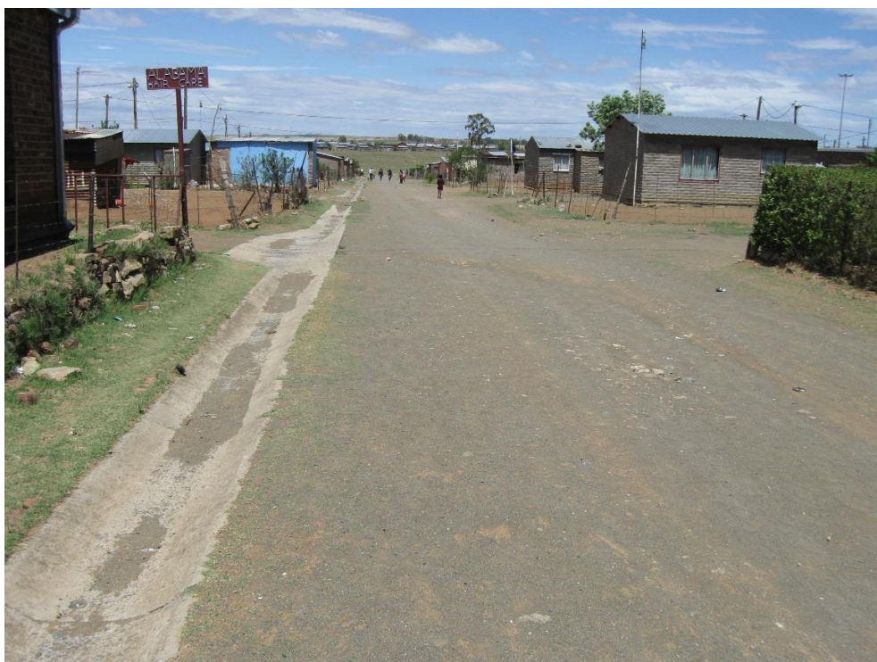
Photograph 5: Gravel street in Roleleathunya. The road is not properly shaped so the channel does not drain the road effectively – grass grows where the water ponds.
