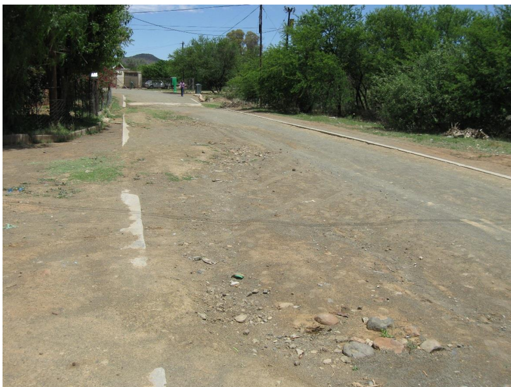
Photograph 2: Proper shaping of gravel roads and channels is required in Mofulatshepe and Rietpoort. Channels should preferably be lined.
