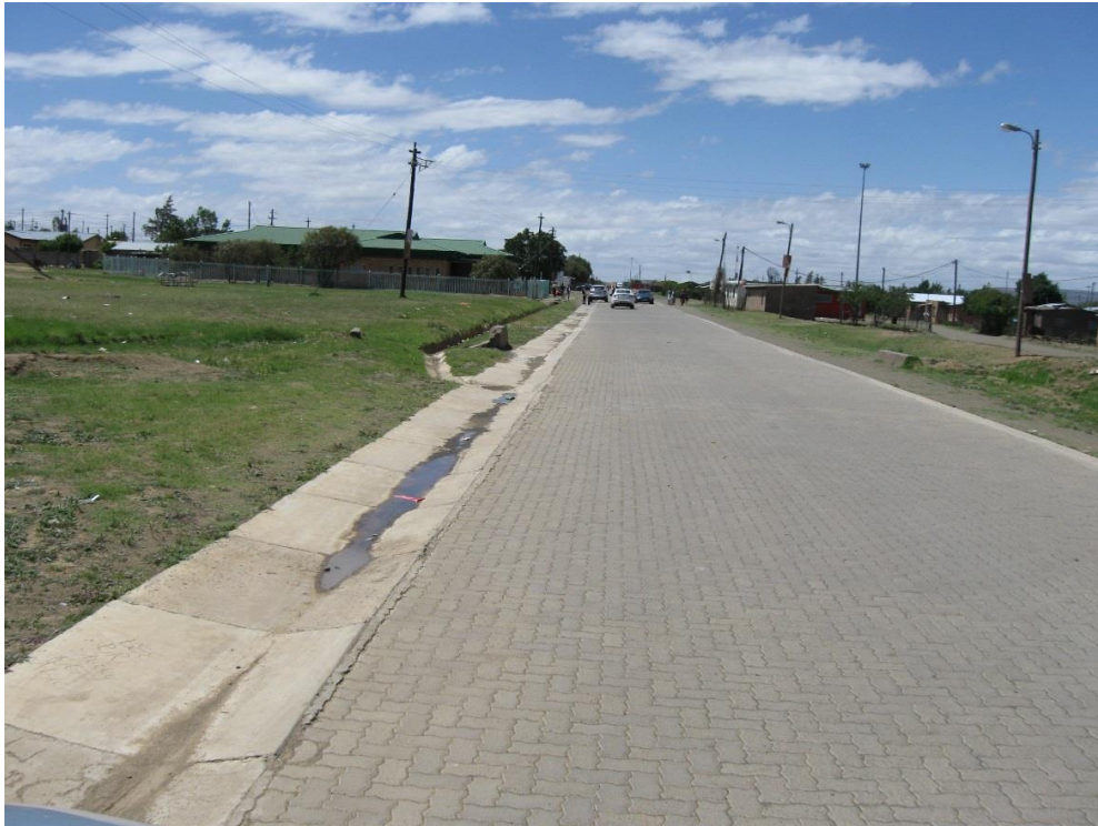
Photograph 6: Posholi Street in Roleleathunya is constructed of concrete block paving and is in very good condition. This type of construction is recommended.
