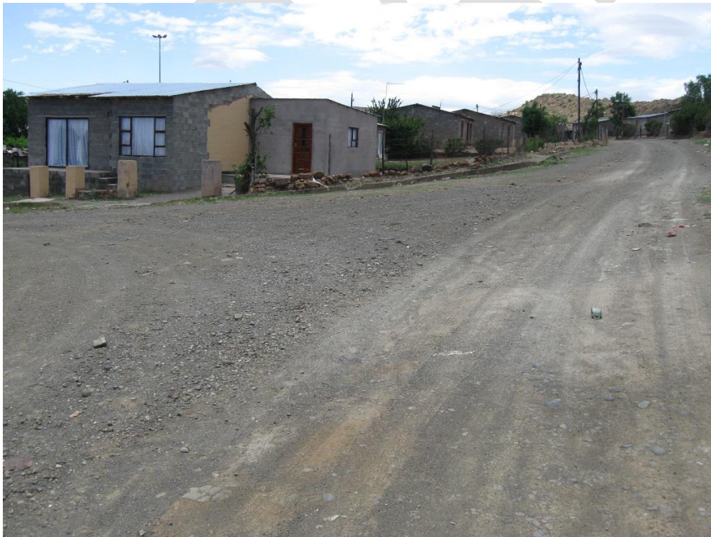
Photograph 2: Gravel roads on steep slopes are subject to erosion, as this street in Rietpoort shows.
