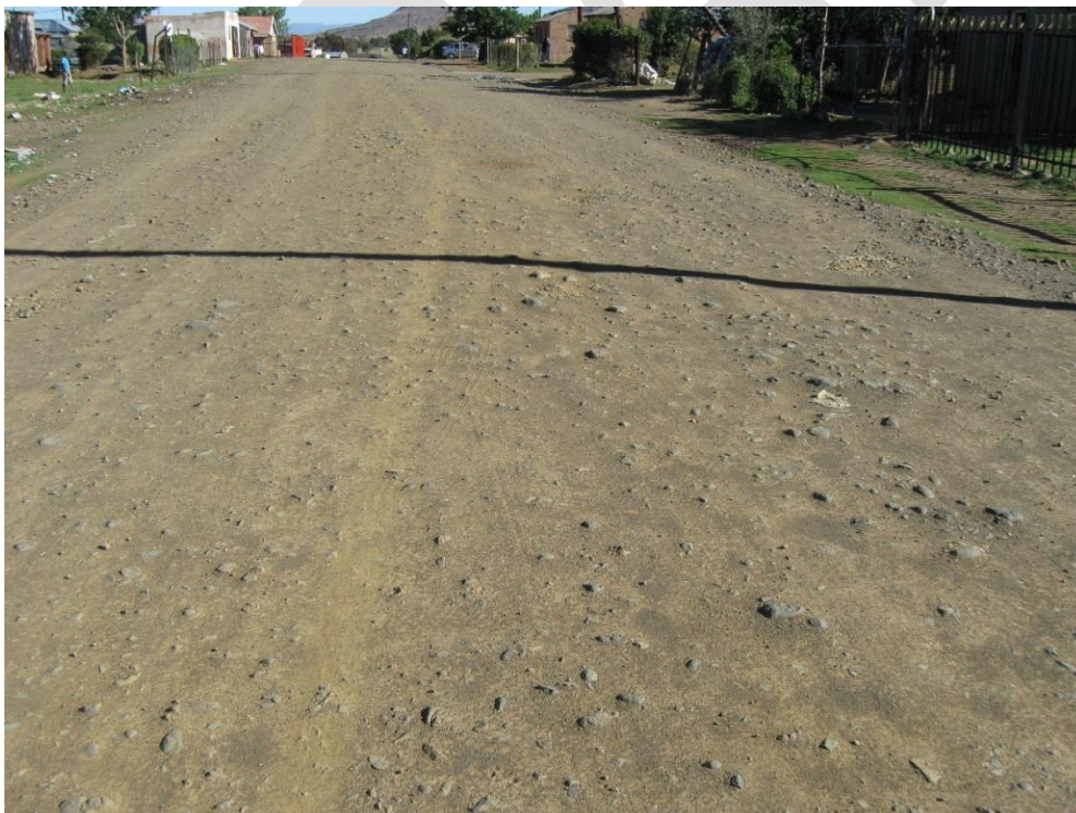
Photograph 14: This is a typical gravel street in Matlakeng. It is eroded and inconvenient for cyclists and pedestrians. Re-gravelling should be undertaken.
